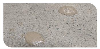
Example: Slightly overfilled mixed material installed into surface spalls.
