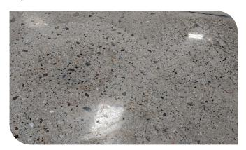
Example: The filled spalls ground flush to the surface and polished up
